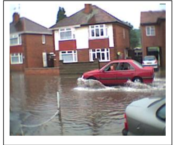
Fig 4 – Flooding in St Albans St, Derby 2001
